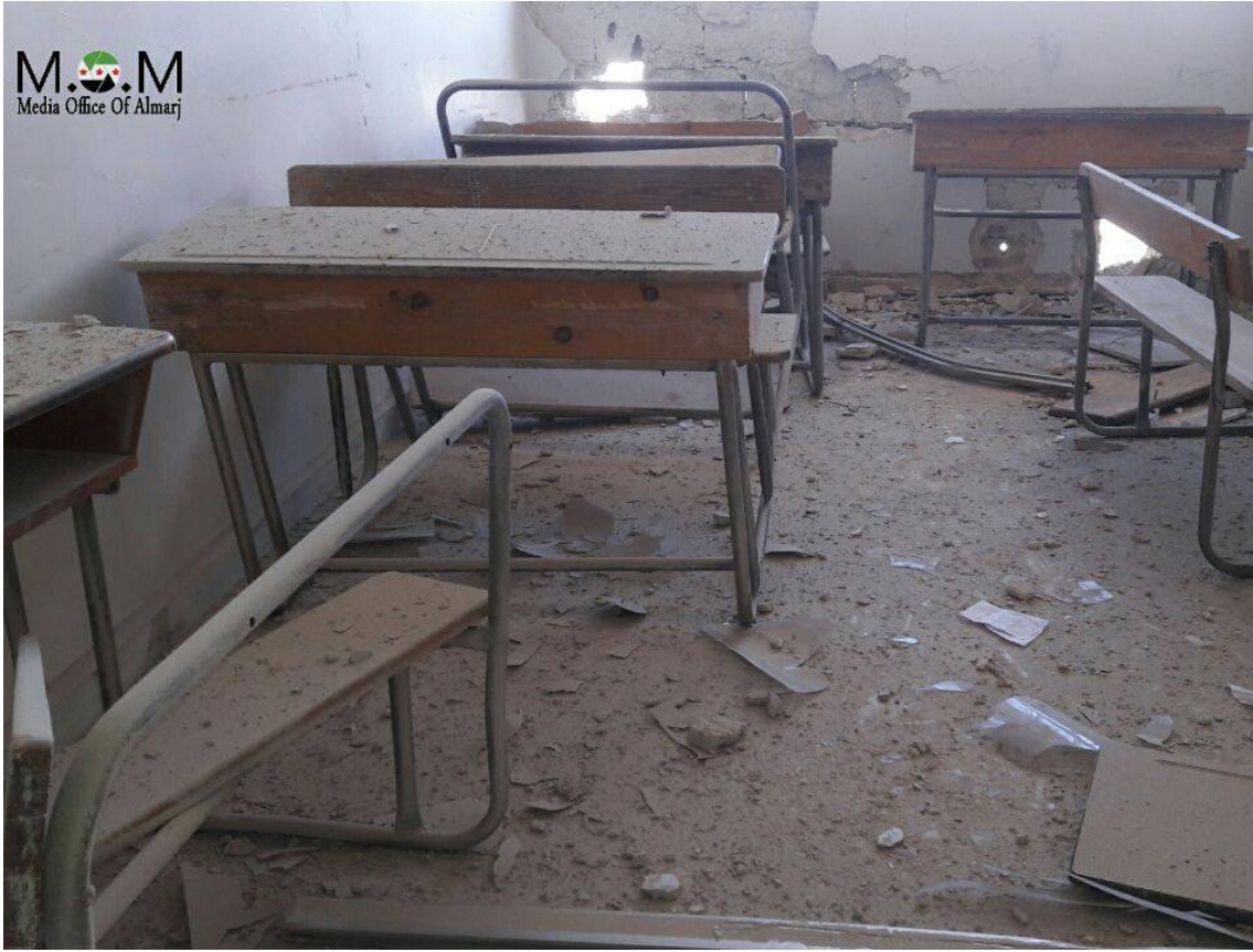
Remains of school in Autaya after airstrikes. 7 March 2017
