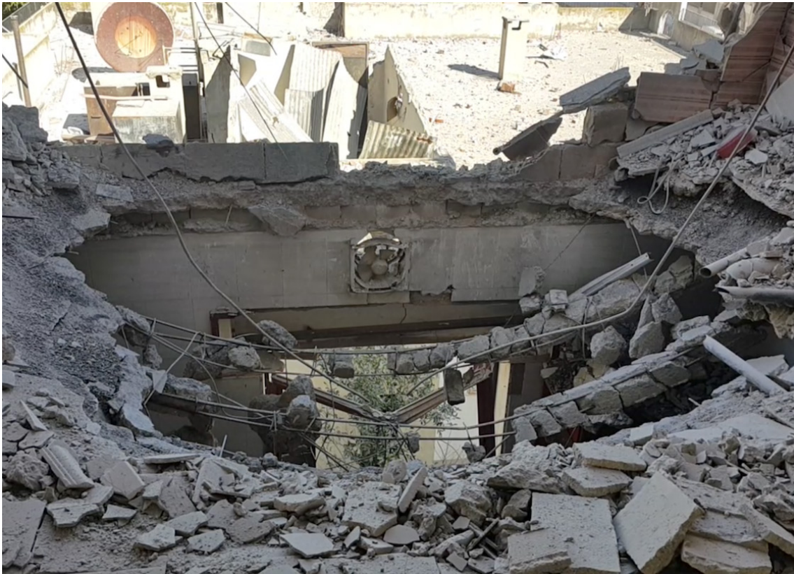
Building damaged in attacks on al-Waer. 17 February 2017
