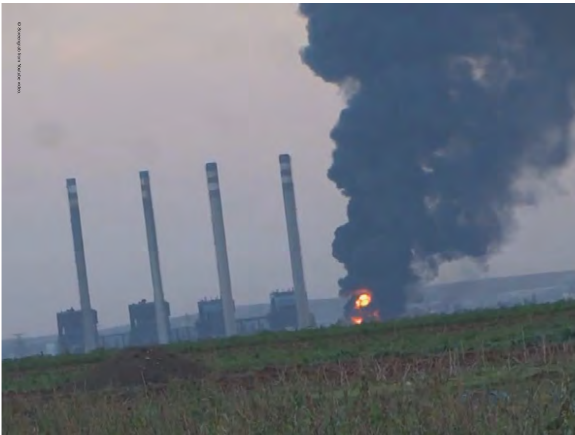
Free Syrian Army rocket attack on the Mhardeh power plant, November 2014.
