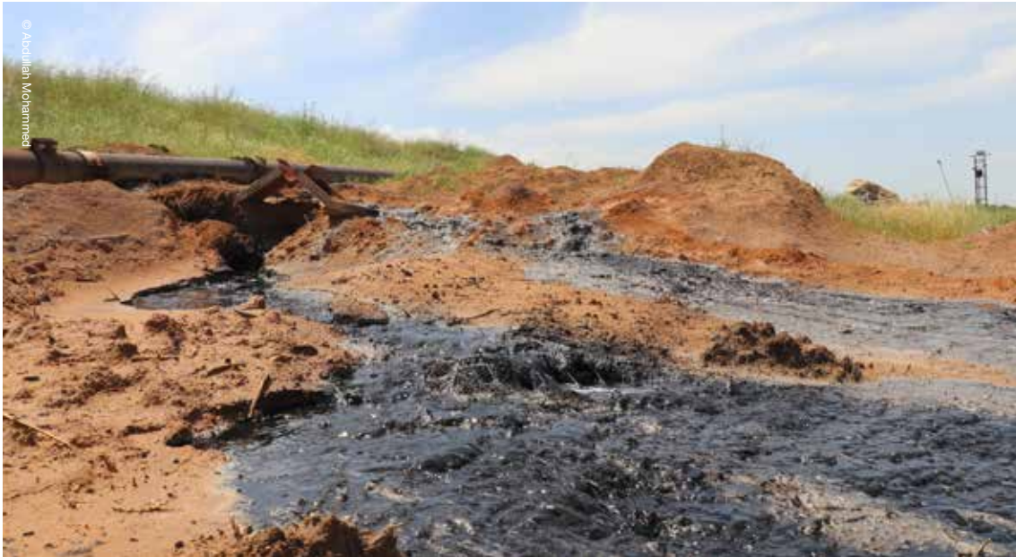
Oil waste flows from a broken pipeline at Gir Zero Oil Facility, April 26, 2020.
