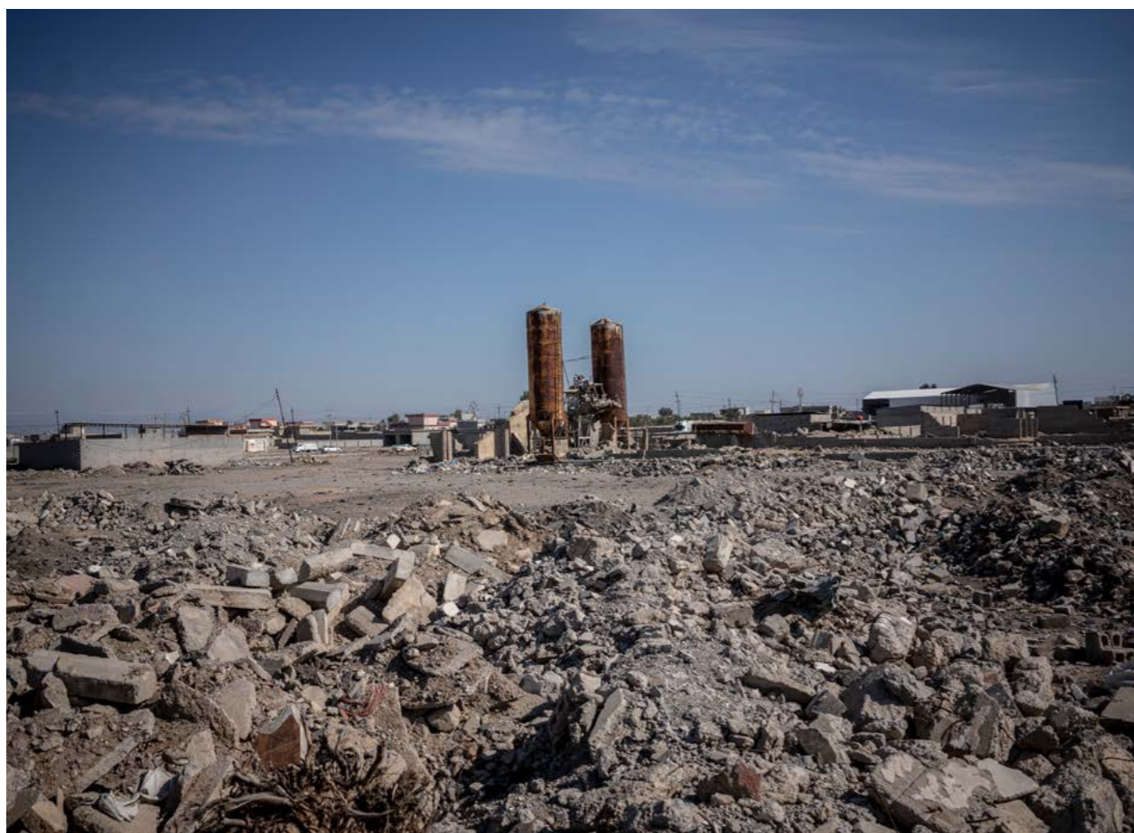
Figure 10: The brick factory which got damaged in the June 2015 airstrike, February 2022. PAX/Ayman al-Amiri.
