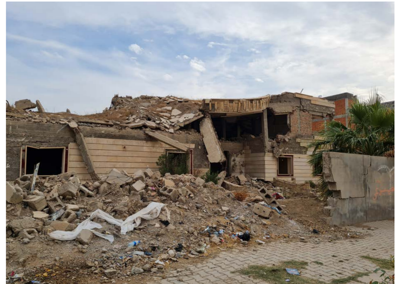
Figure 8: Damaged houses next to the industrial neighbourhood, November 2021. PAX/Saba Azeem.
